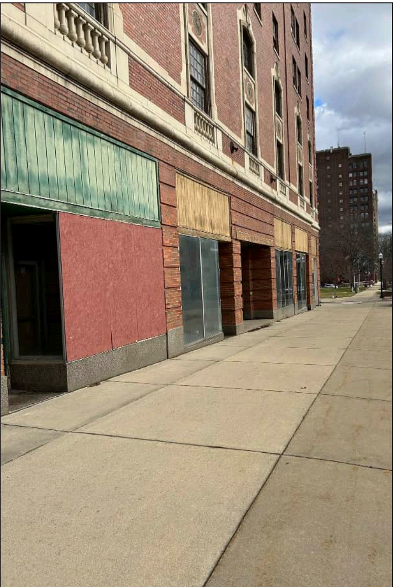
1. S01 - South Elevation, First Floor.
