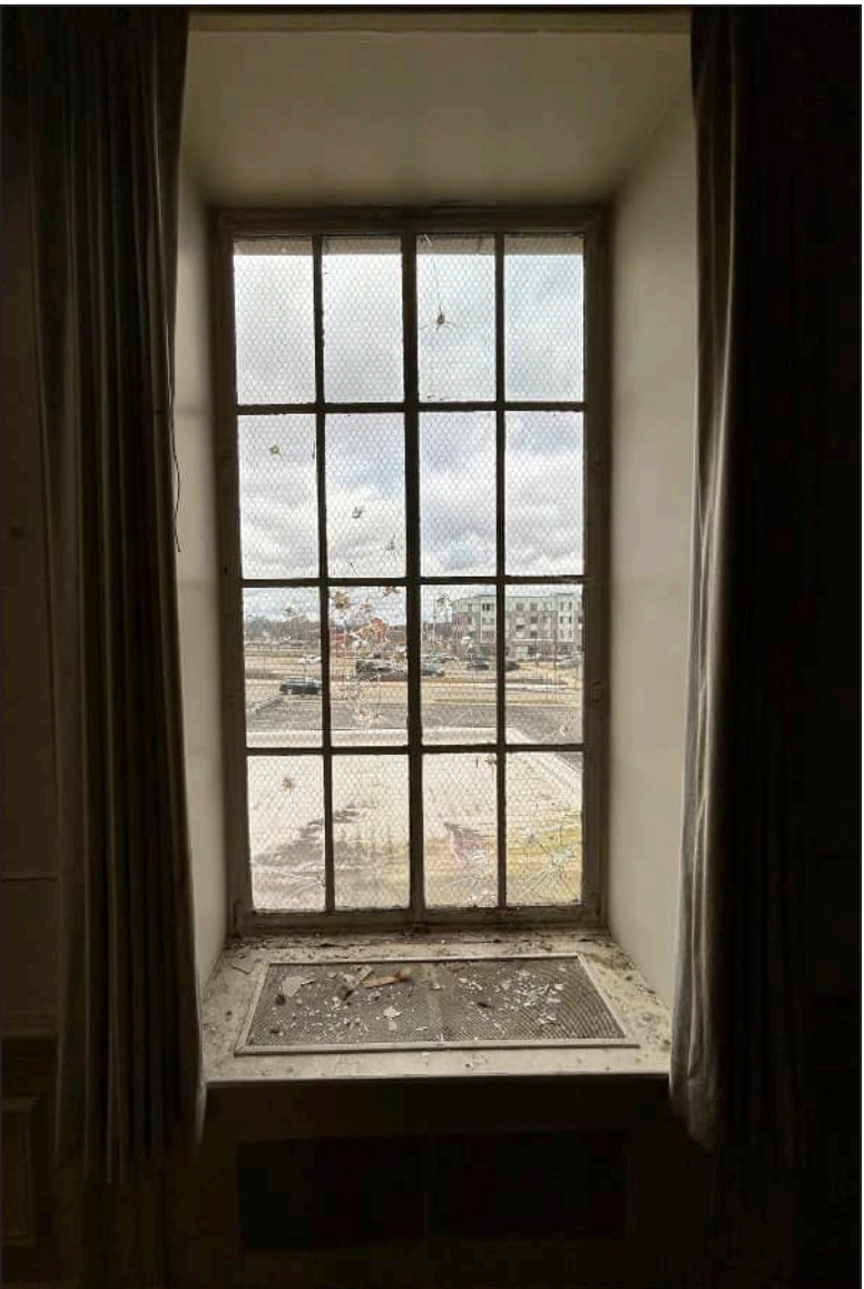
67. N01 – North Elevation, Second Floor.
