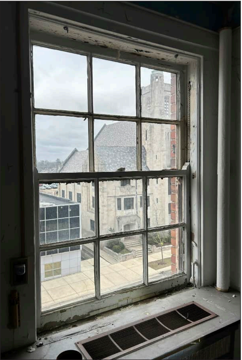
22. S22 – South Elevation, Fifth Floor.
