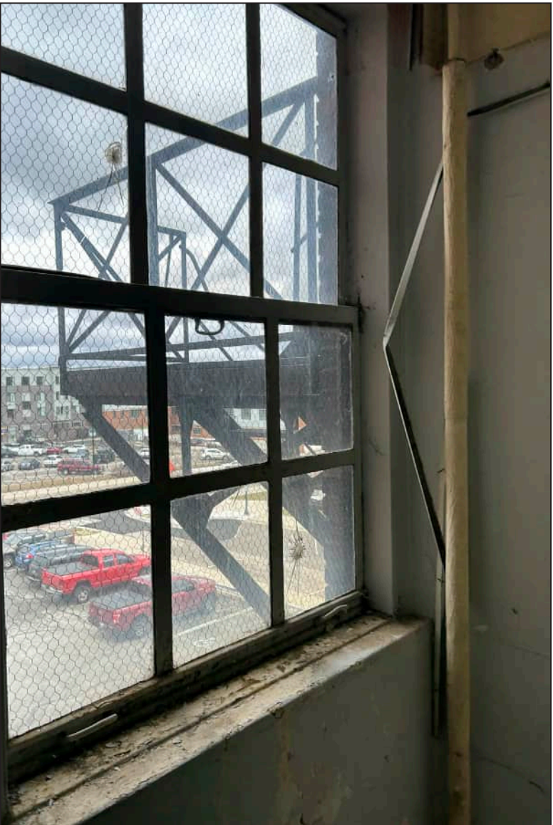
69. N03 – North Elevation, Third Floor.
