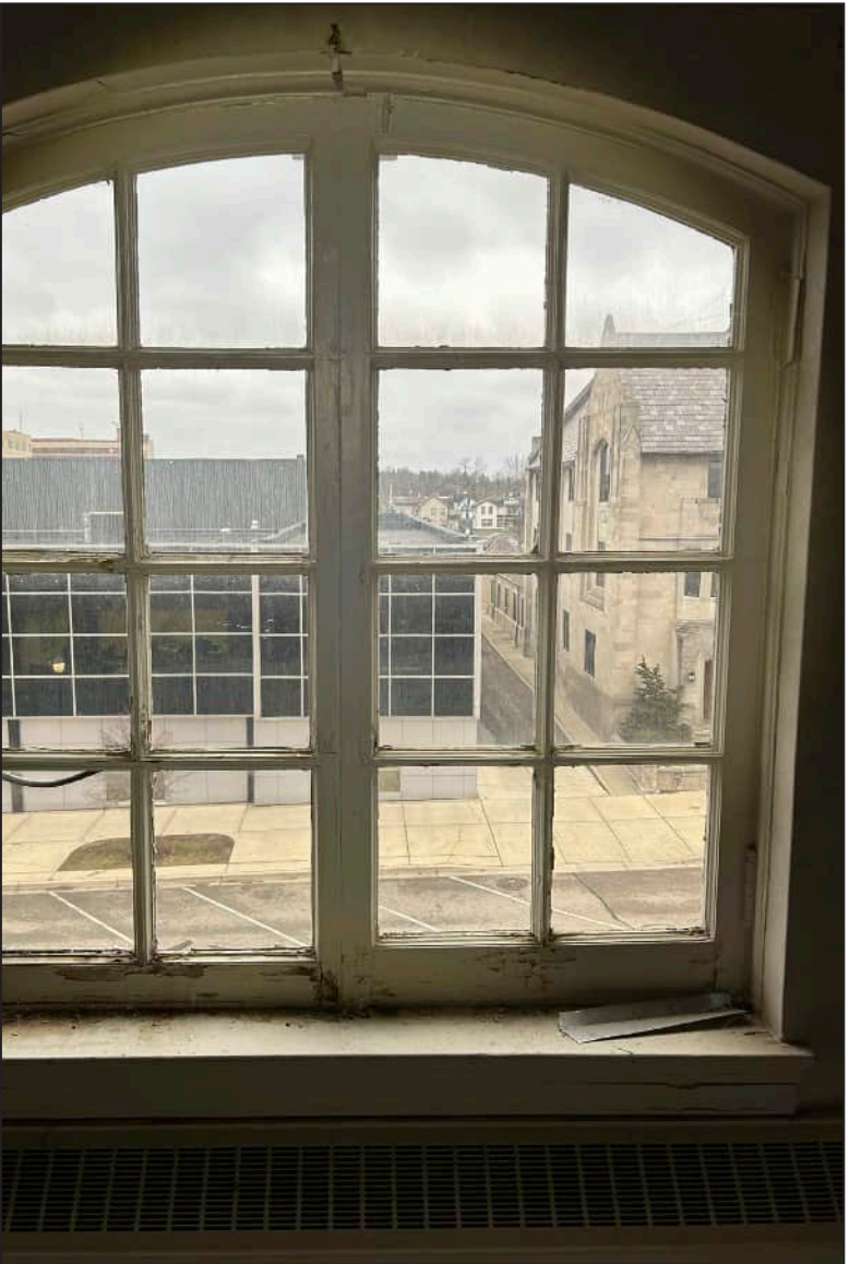
18. S18 – South Elevation, Fourth Floor.
