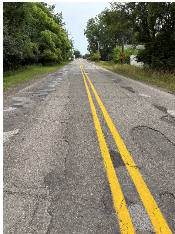
Photo 4: Washington Ave, facing west from west of Elm
