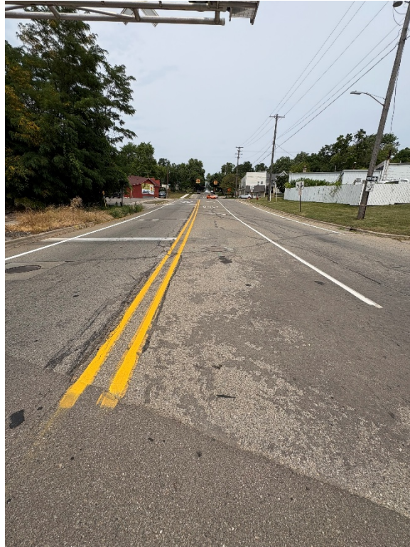
Photo 3: Elm Ave, facing north from slip ramp
