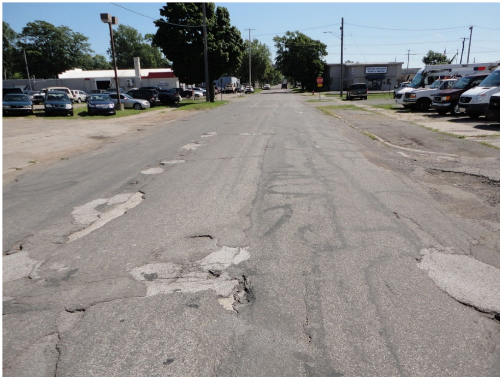
Photo 2: Pearl Street mid-block between Cooper and Pearl looking east
