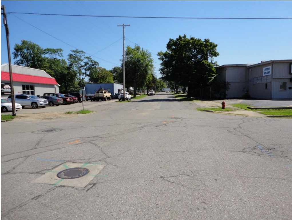
Photo 3: Pearl Street at Park Avenue looking east
