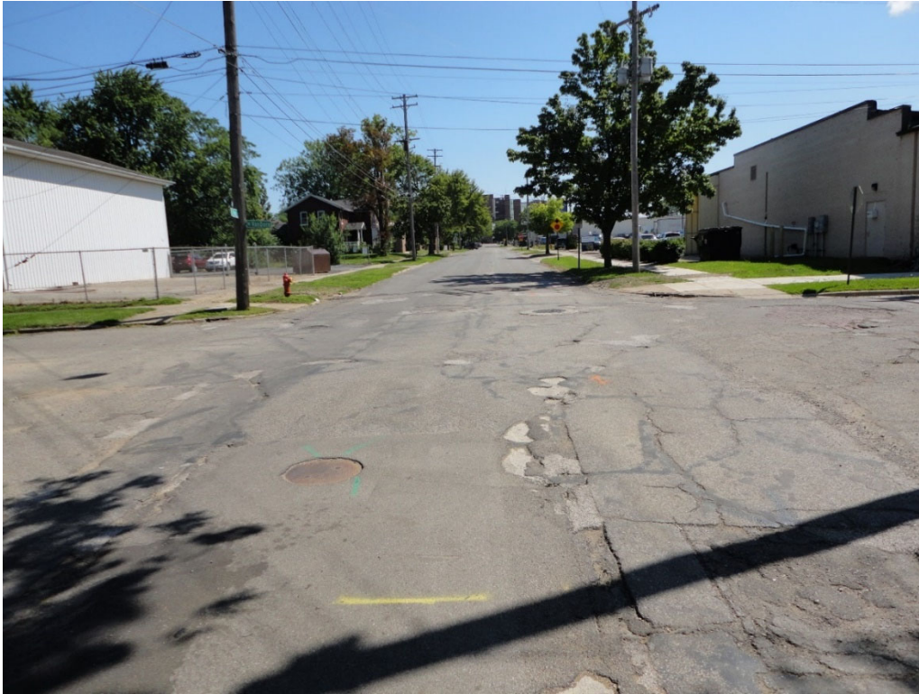
Photo 5: Pearl Street at Van Dorn looking east
