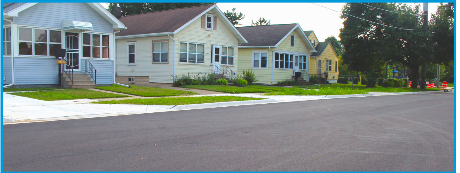
Reconstruction project complete on Blakely Avenue.
