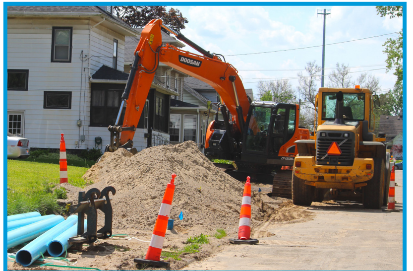
Water main replacement on Arnold Street.
