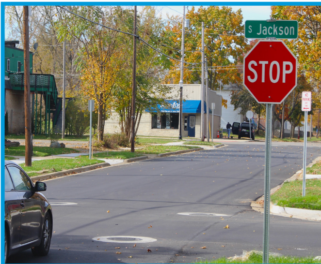
Construction project complete on W. Biddle Street.
