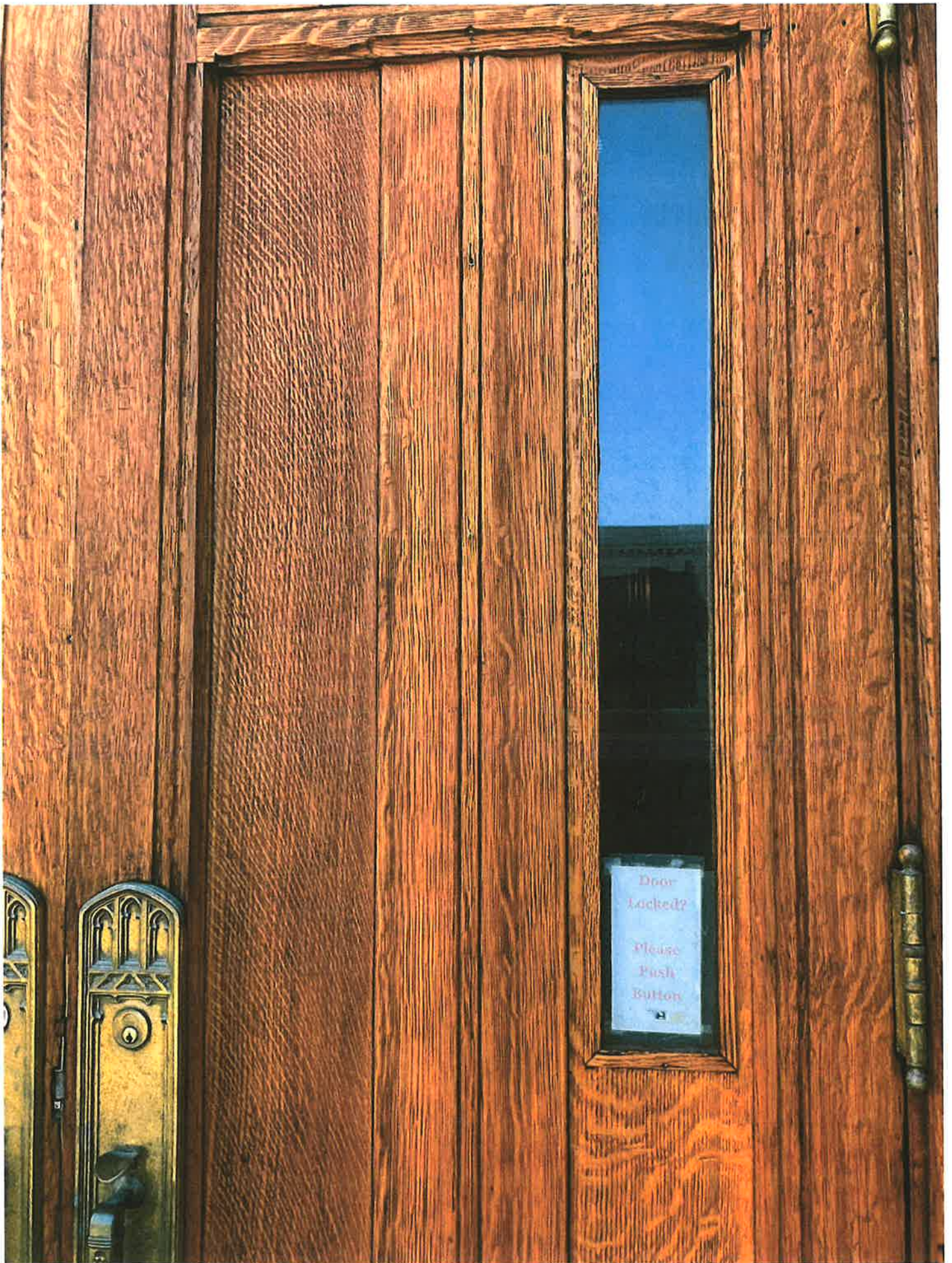
Close Up of Existing Window
