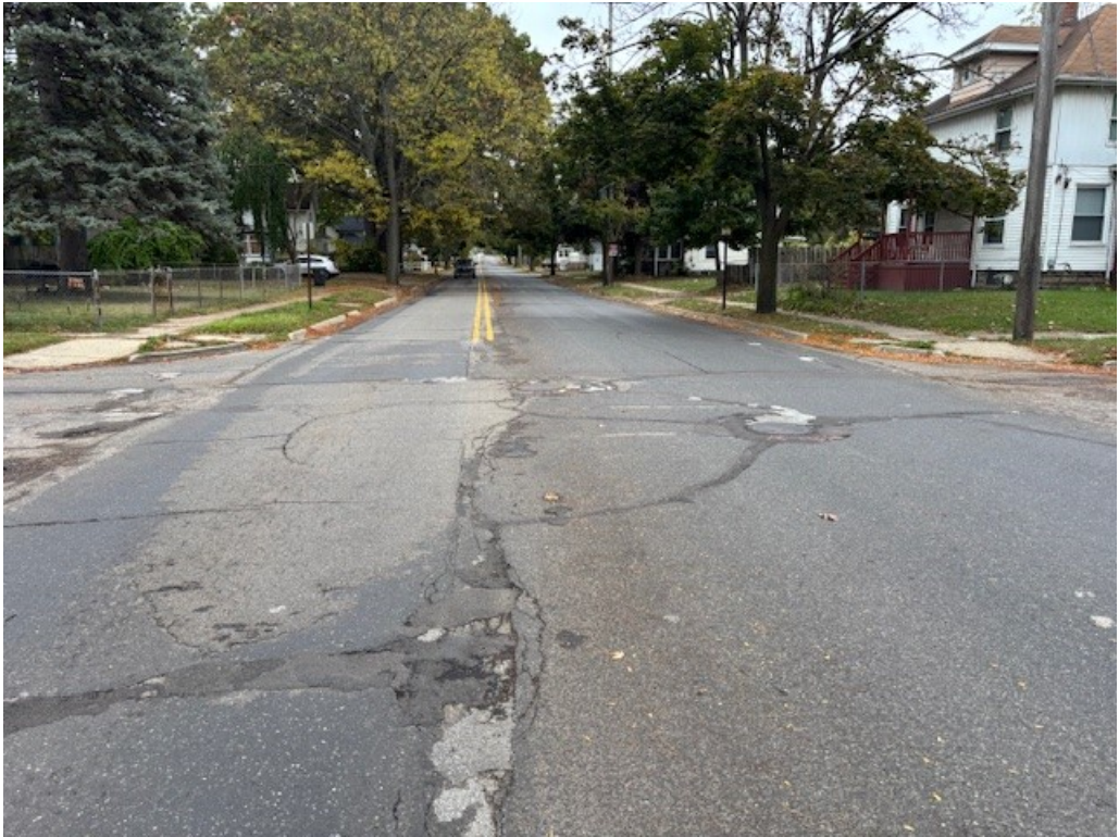
Photo 3: Ganson Street, facing east from Bates Street intersection
