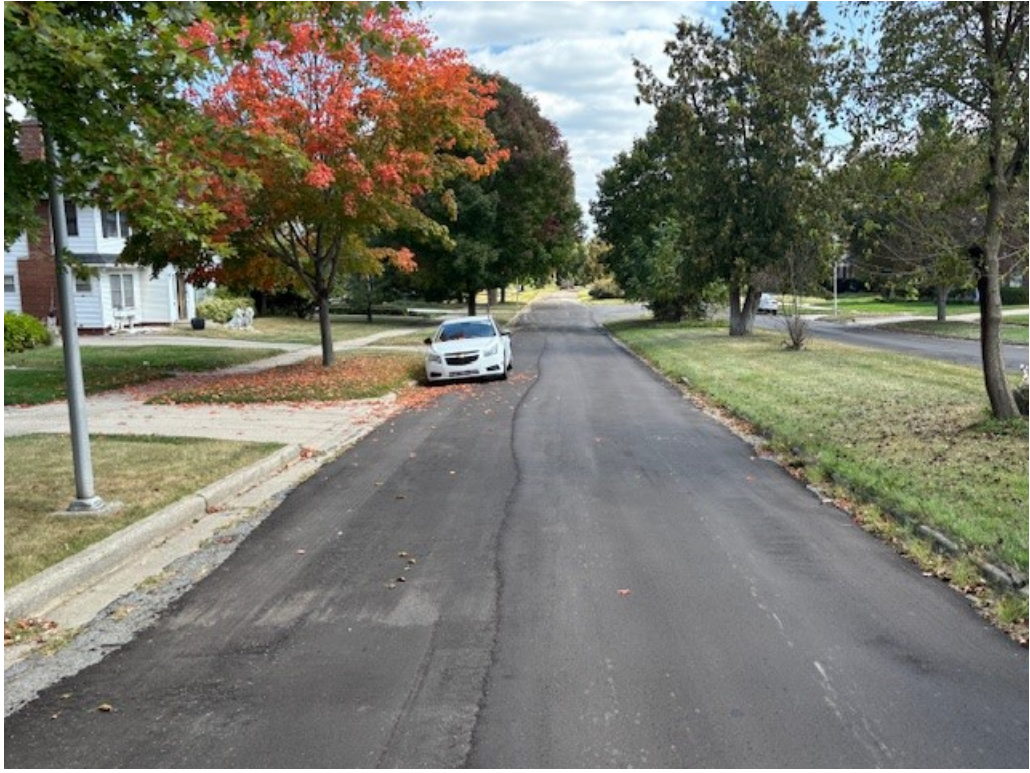
Photo 2: Facing east in the north lane in front of 754 Bloomfield Blvd
